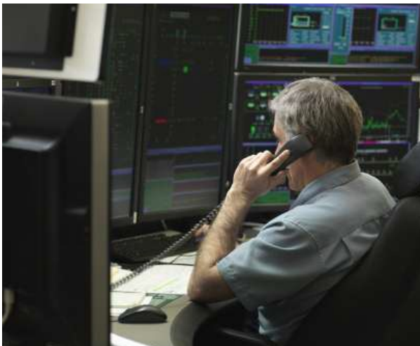
Pipelines, including Line 5, are monitored around the clock by operators in our state-of-the-art control center
