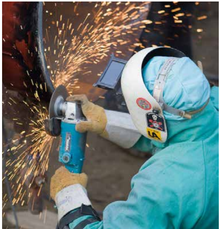
Welder is conducting pipeline repair as part of Enbridge's Integrity Management Program.
